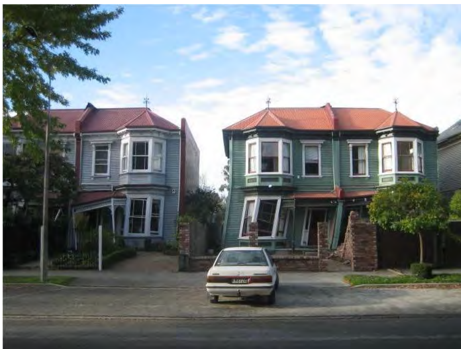
An example of a “soft-storey”. Photo: Des Bull, Holmes Consulting
