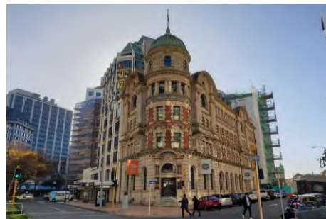
The former Public Trust Building (1909) was designed to resist fires and earthquakes. It was earthquake-strengthened in 2015. Photo: Moira Smith.
