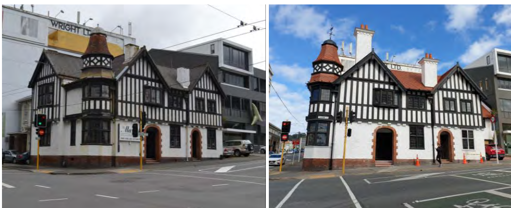
The chimneys at 200 Willis Street have been reinstated as lightweight replicas. Photos: Wellington City Council (left) 2015 and Moira Smith (right) 2023.
