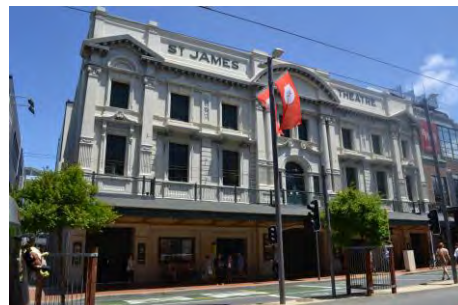
The St James Theatre (1912) re-opened in 2022 after earthquake strengthening. Photo: Wellington City Council.
