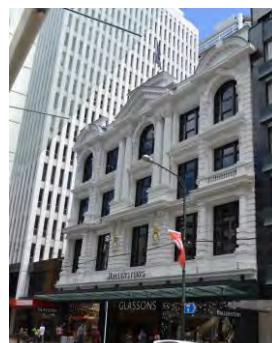
Many decorative parapets and clocktowers were removed from Wellington buildings in the 1930s and 40s. The parapet at the Whitcull's Building (1907) was removed in the 1930s, and later restored as a replica. Photo: Wellington City Council.
