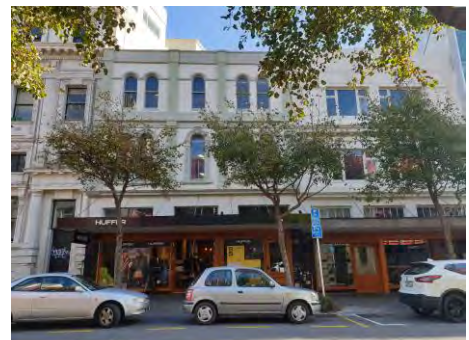
The former T.G. Macarthy Trust Building (1897-1904) was strengthened in 2018 with help from the Built Heritage Incentive Fund (BHIF). Photo: Moira Smith.
