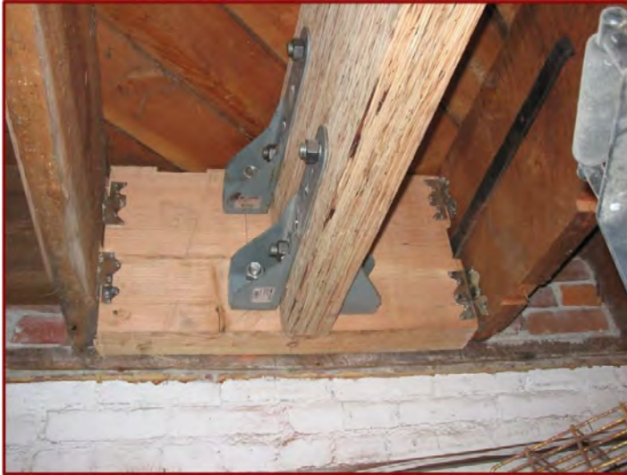
Examples of a detail for anchoring walls to the floor diaphragms. Photo: Lara Simmons
