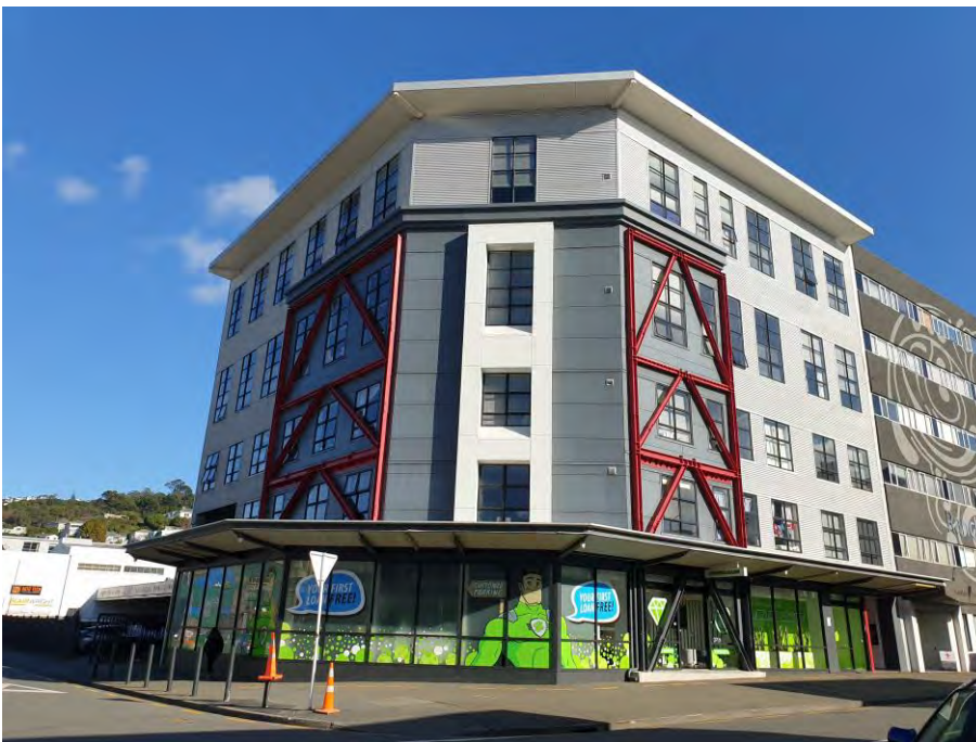
This is an example of external structure known as an “exoskeleton” on the exterior of a non-heritage building. Photo: Moira Smith.
