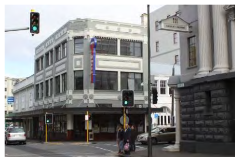
Morgan's Building (1922) was strengthened in 2012 with help from the BHIF. Photo: Wellington City Council.
