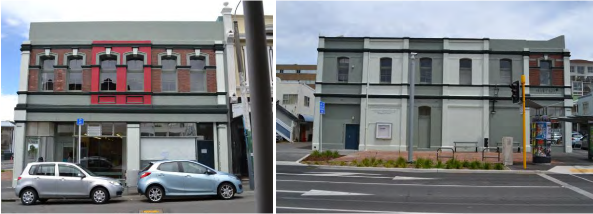
Cuba Street's Thistle Hall is a good example of sympathetic works to strengthen a heritage building.
