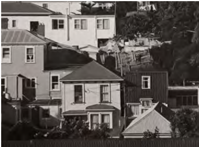
The A-framed addition under construction in 1977. No.125 is to the left.
