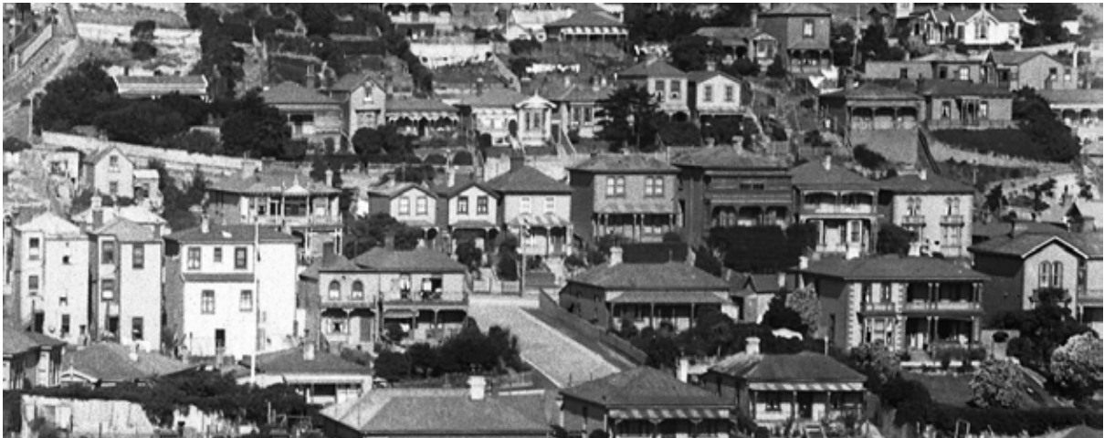
Part of lower Hawker Street, about 1910, before major changes were made to the houses. Duke Street, a no exit street off Hawker, is in the foreground. (1/1-022833-G, Alexander Turnbull Library)
