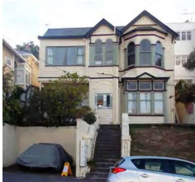
The house in 2016. The most obvious changes are the infilled first floor verandah (and part of the ground floor verandah) and the loss of decorative detailing.
