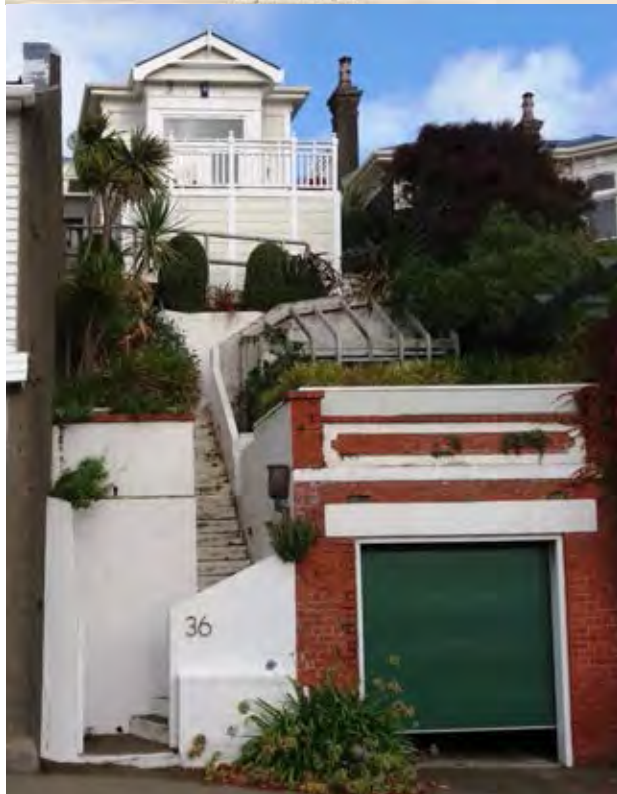
36 Hawker Street – 1904 alterations above (WCA) and, pictured in 2017. (M. Kelly)
