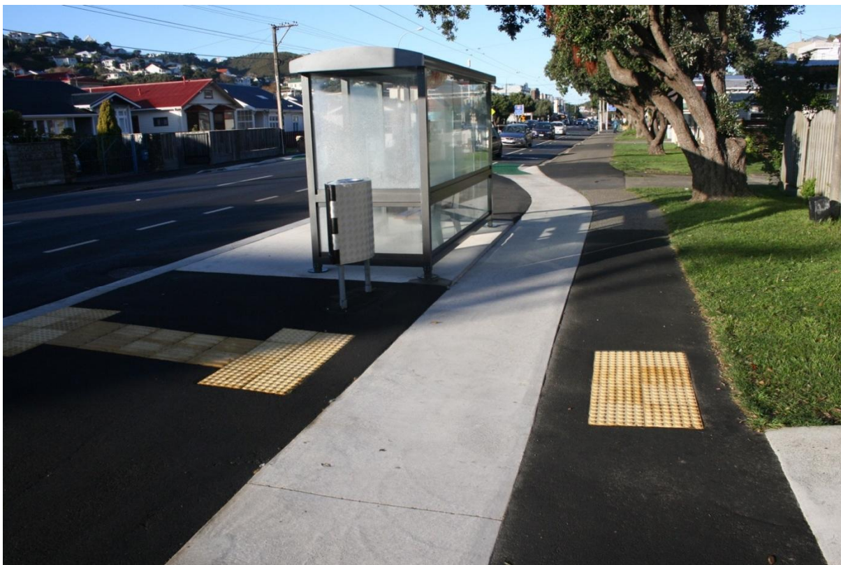
Image showing pinch point in footpath width at bus stop along the Parade
