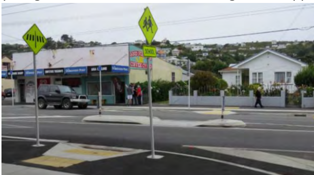
The “Safer Route” crossing
