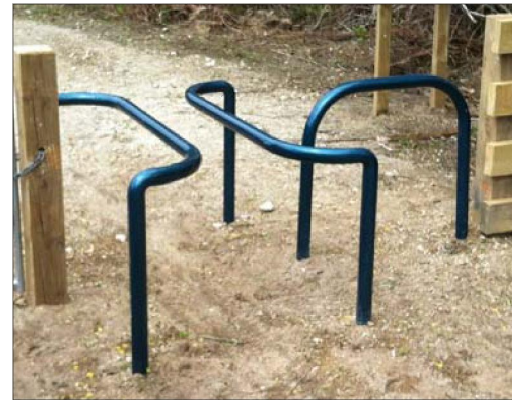
A PHOTOGRAPH OF SQUEEZE BARRIER IN SITU. 001 Not to a particular scale
