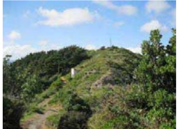
Telecommunications tower on the ridgeline
