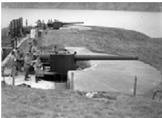
1937 photo of original 6-inch gun emplacements positioned facing south over the harbour entrance.
