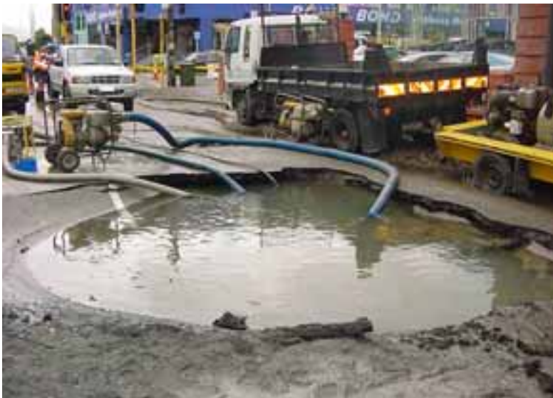
Tory Street 450mm water main burst
