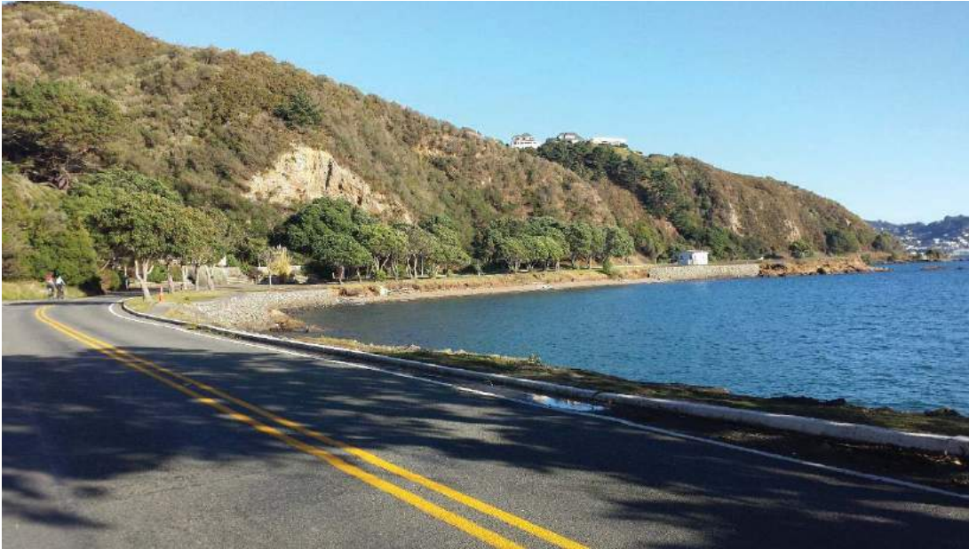
Southern bay showing various sea wall treatments
