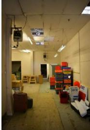
Fig. 80 View of a typical room in the single storey section of the building. Note the plain sheet linings on walls and ceilings.
