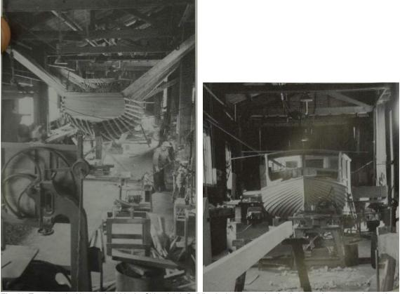
Fig. 19 Two views looking north within the Shipwright's Building in the 1950s, showing boats under construction and repair. Note the monopitched roof, with half-truss roof structure. (Berthold, "B.T. Daniel Ltd., Shipwrights, Boatbuilders & Marine Engineers, Shelly Bay, Wellington," *New Zealand Marine News* v.58, no.1, p20)
