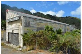
**Fig. 57** View towards the north western corner of the Shipwrights' Building. Note the large timber swing doors in the north gable end.
