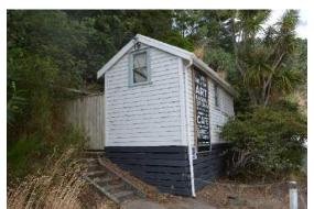
**Fig. 64** View of the outbuilding looking towards the west gable. Note the concrete steps which provide access up to the main entrance and the shiplap weatherboards on this gable.
