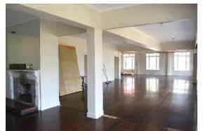
**Fig. 40** Looking south east at ground floor level towards the central room partition which features the fireplace mantle and hearth. Note the timber floors and window joinery..
