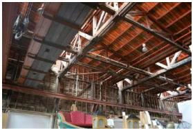
Fig. 89 Interior view looking west across the high stud double storey section of the building. Note the timber roof structure with wide span ladder trusses, heavy gauge structural timbers, exposed purlins and sarking.
