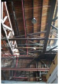
Fig. 86 View of the timber roof structure. Note the wide span ladder trusses, heavy gauge structural timbers, exposed purlins and sarking.
