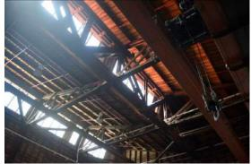
Fig. 90 Looking back towards the south aspect. Note the glazed portions of the saw-tooth roof profile.
