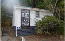
Fig. 65 View of the outbuilding looking towards the south elevation. Note the concrete steps which provide access up to the main entrance and rusticated weatherboards on this elevation.
