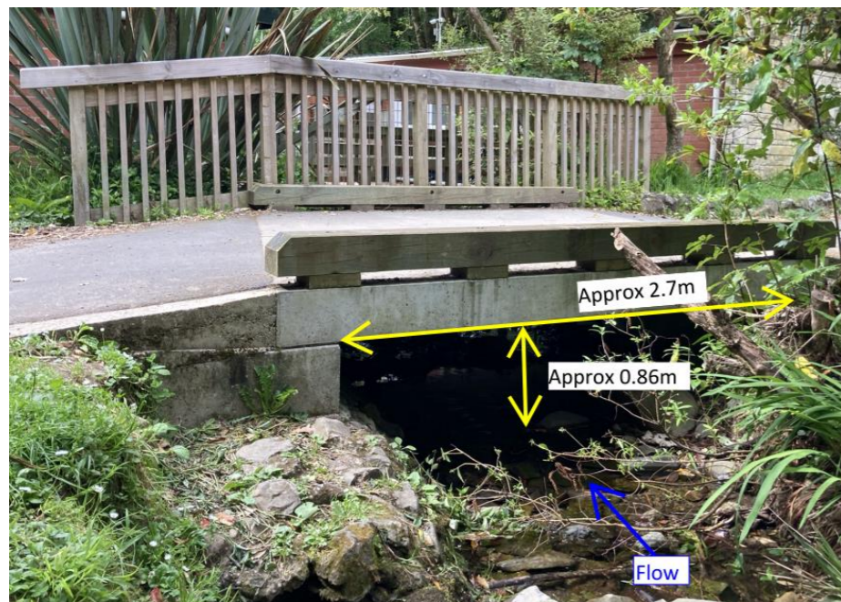
Figure 2.3 Existing footbridge and Tyers Stream located to the west of the site.
